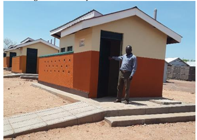
The head teacher shows one of the 5 stance latrine blocks constructed by ACORD with funding from HEKS
