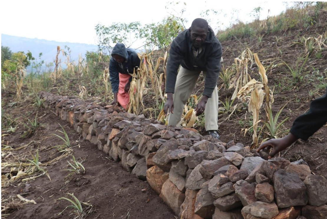
Photo: Community members constructing a stone band in Kamukaki micro catchment
