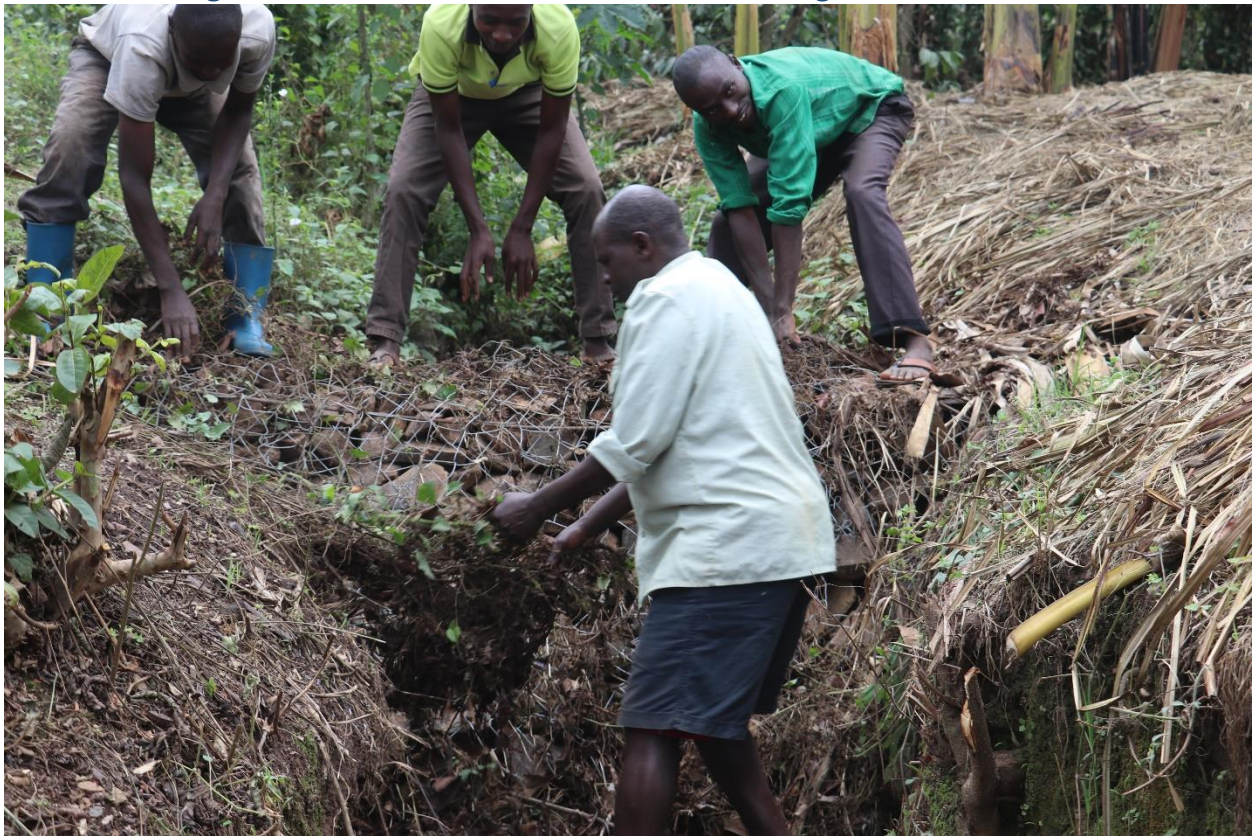
Photo: Ihoho Community members Rehabilitating a gabion
