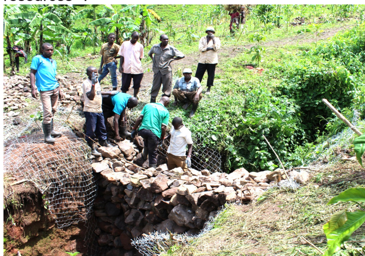
Construction of Gabions for Gully rehabilitation
