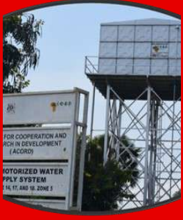
One of the Water Supply Systems constructed by ACORD U with HEKS-EPER financial support in Zone 4 Bidibidi refugee settlement, Yumbe District. © Romeo
